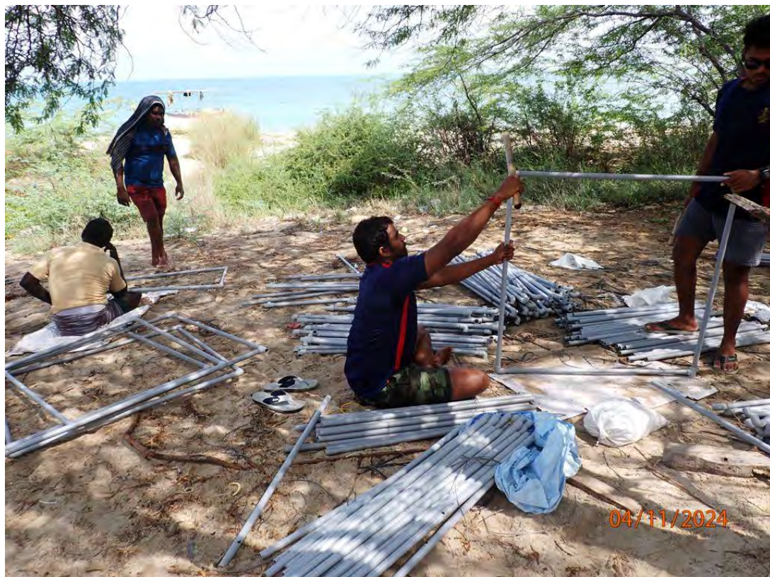
Fig.14: Construction of PVC frames in the field
